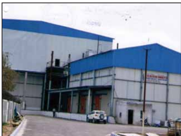
M/s R S Freezing &amp; Cold Storage Pvt. Ltd., Kundli (CA Store)
